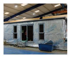
Protect VC Foil Ultra – this reflective and low emissivity air and vapour control layer was used on the warm side of the insulation within an unventilated cavity. Combined with Protect TF200 Thermo, this helped the structure achieve its target thermal performance.
