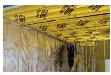
Protect sealing tapes – these were used with the above construction membranes to ensure correct detailing in the sealing of overlaps to significantly reduce air leakage and therefore keep energy consumption to a minimum.
