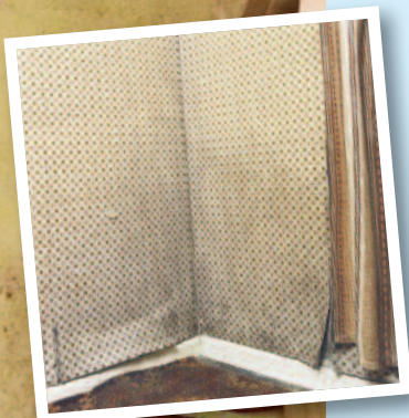
Photographs to the left show the results of harmful condensation.
