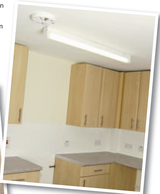
A161 humidity-sensitive extracts in kitchen and bathroom
