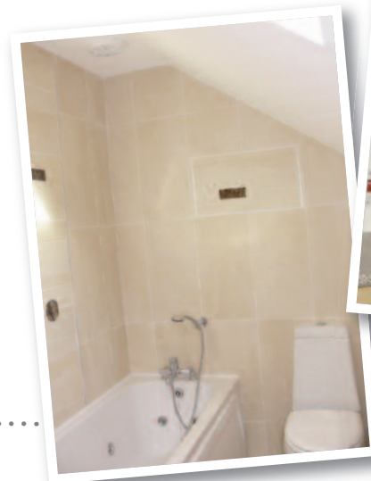
A161 humidity-sensitive extracts in kitchen and bathroom
