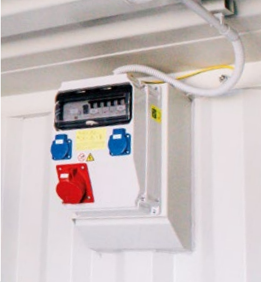
Distribution box with integrated sockets
