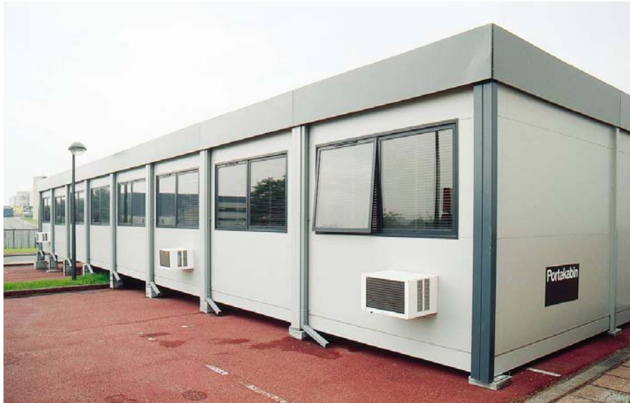
Figure 4.1 An example 8-module building (with air-conditioning) which relates to a generic 10-module building used for the notional building.
