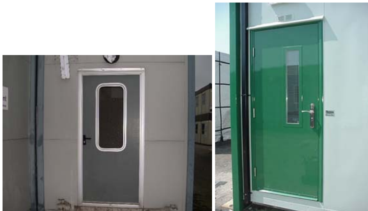
Figure 3.3 Upgrade of old to new doors.
