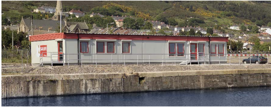
Figure 2.3 7-module building (Swansea Docks).
