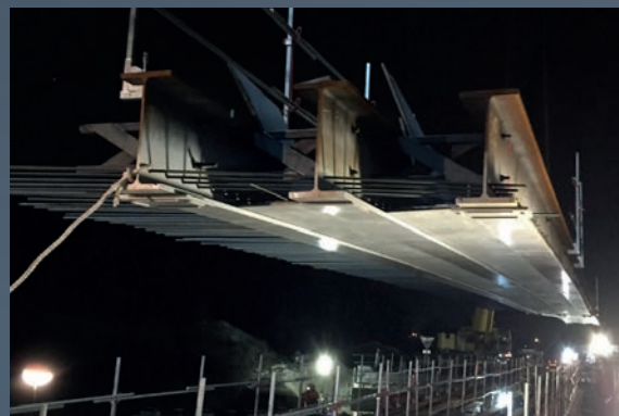
A75 AUTOROUTE France
