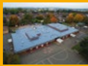
LIQUID APPLIED ROOFING
