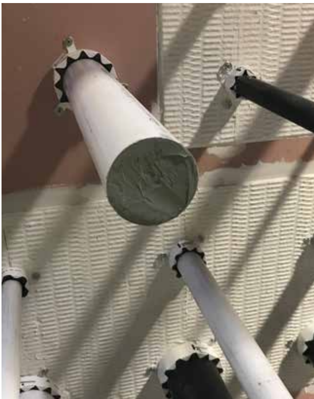
Pipe collars before ...
